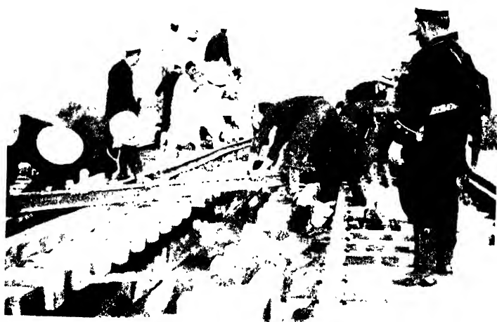
REPAIRING THE LINE.
